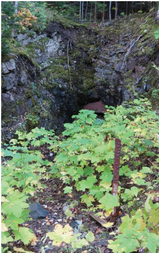
Figure 7. A gated adit entrance to part of the underground workings of the Petherick mine, with a modern site marker, engraved “Petherick Shaft” in the foreground.
