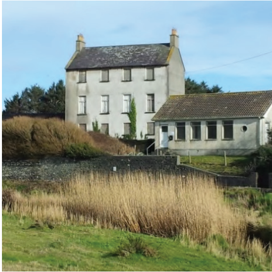
Figure 8. The semi-derelict, 3 storey over basement house, Bunmahon, Co. Waterford known locally as "Petherick's house". It was built in the 1840s and served as the home of John Petherick for much of the time while he was employed by the MCI.
